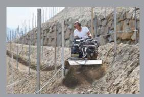
with a mini excavator, screw conveyor or spider excavator. Terracing with a mini excavator is slower, but leads to more compact and stable terrain and the embankment can be shaped immediately. Terracing with a screw conveyor takes less time, but then the resulting "nose" must be removed by hand
